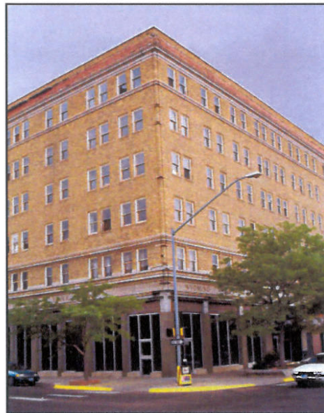
The historic Wyoming Building Downtown, is both an asset and liability, but a critical resource.
