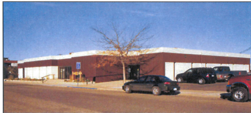
The Natrona County Health Department recently moved into these offices in the West Central Corridor.
